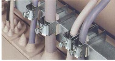
Figure 5-2. Strain Relief Clamps in the Cabinet
