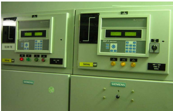
The two EGCP-3 MCs were installed in the main switchgear cabinets
