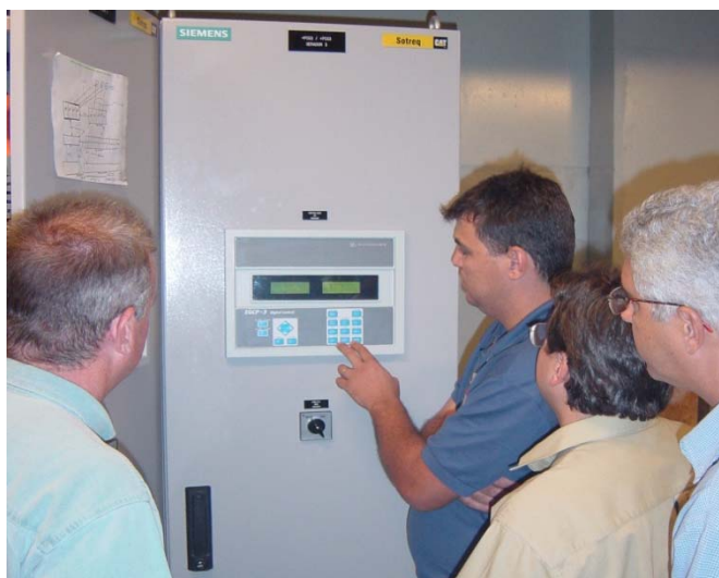
Configuring one of the EGCP-3 LS units via the front panel
