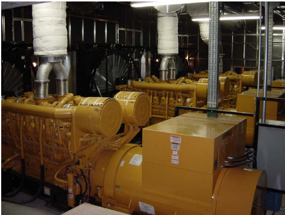
Three EGCP-3 LS units were used to control the three Caterpillar gen sets
